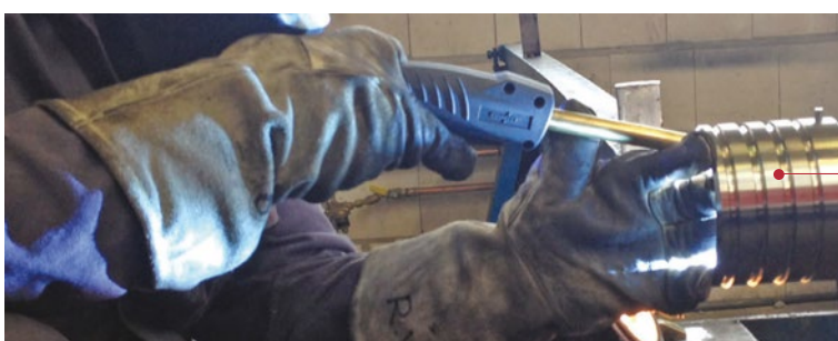
Welding inside pipes with extra long torch neck and small bend radius
